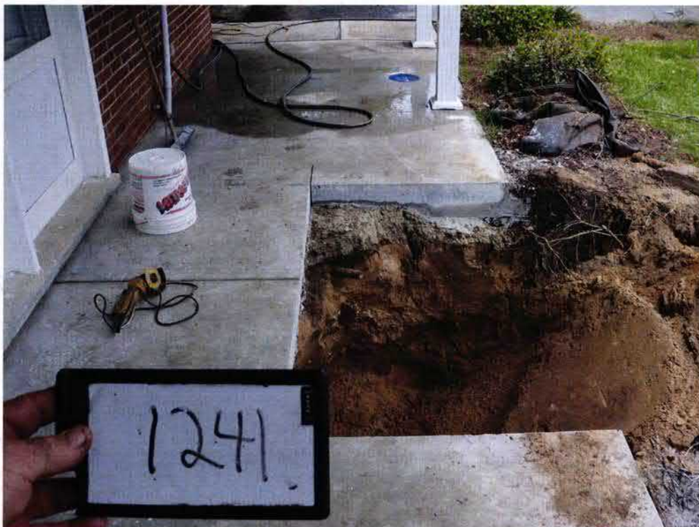
Picture 2: UST 1241Dove excavation.
